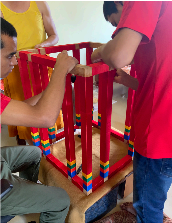
3. The skeletal interior foundation of the Abode that will hold the structure of the Substitute Abode
